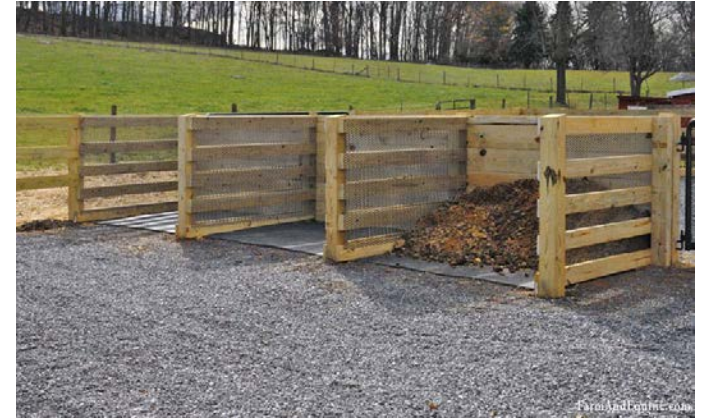
Above: A three-bay compost bin system on a gravel pad.
