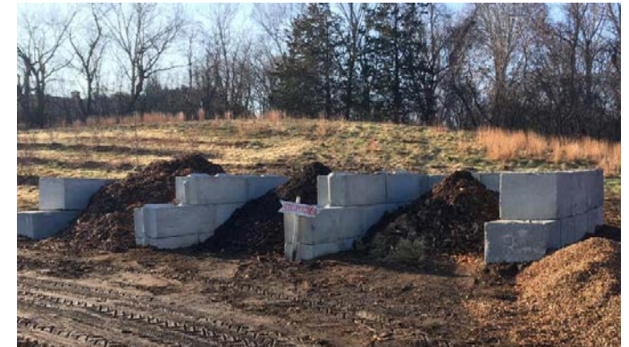
Above: A three-bay compost bin system using concrete blocks instead of lumber.
